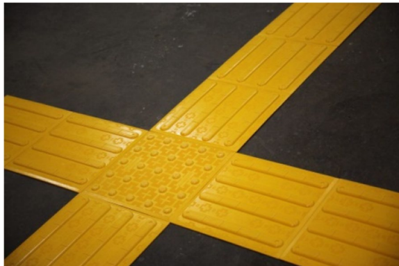
Fig. 12 Wayfinding tiles on the roads designed for blind people. (Source: www.tactilesolution.ca )
